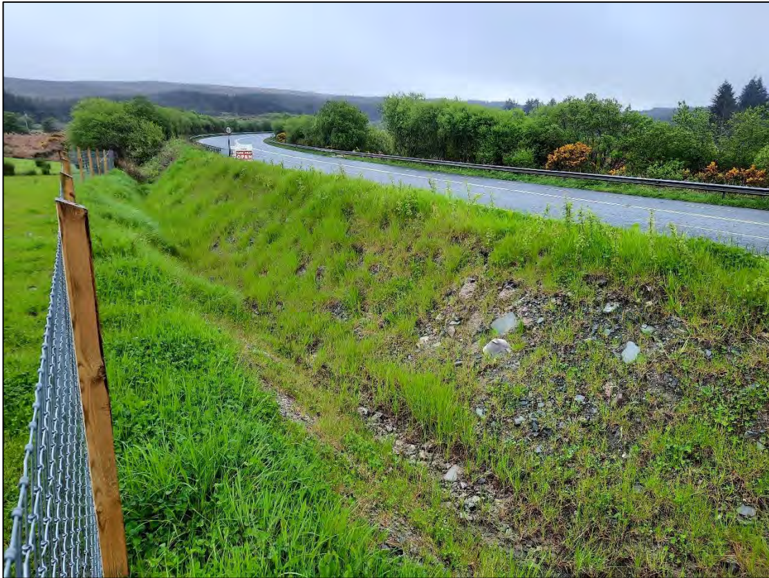
Plate 2- 39 View of dry Drainage ditch (FW4) located within the footprint of the proposed temporary access road off the N22 associated with the TDR.
