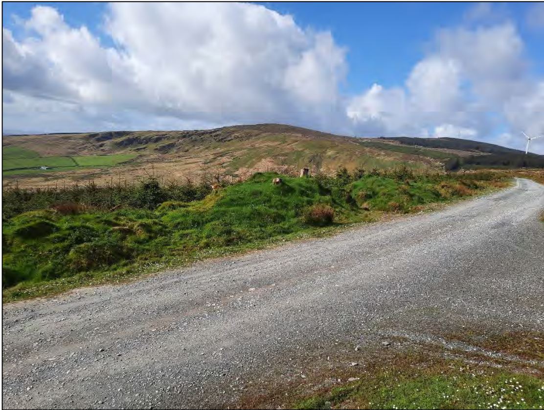
Plate 2- 6 View of forestry roadway classified as Buildings and artificial surfaces (BL3) and surrounding Dry Meadows and Grassy Verge (GS2) habitat into which the 110kV cabling will be laid.
