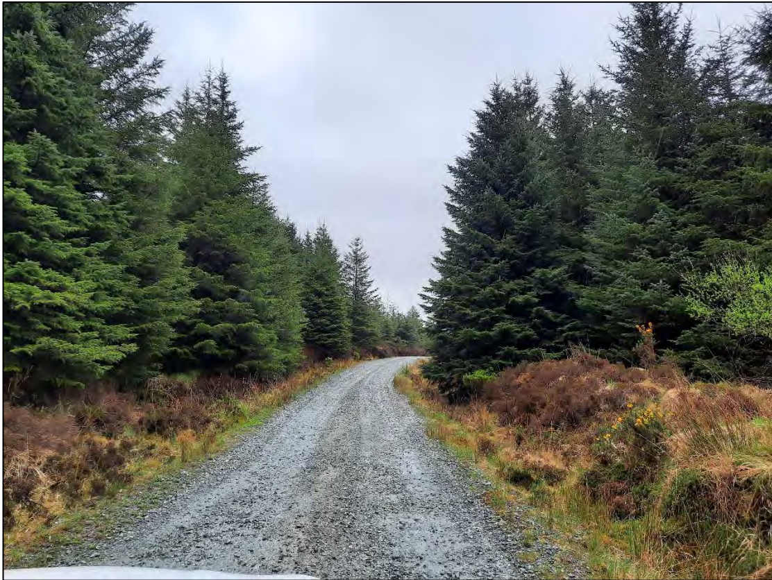
Plate 2- 27 Typical view of forest roadway classified as Buildings and artificial surfaces (BL3) located within the footprint of the proposed TDR works.
